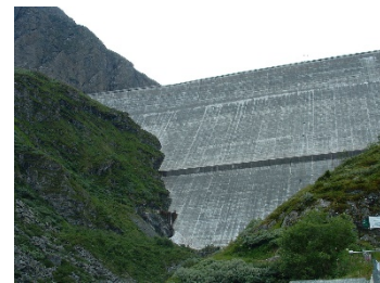
Grande-Dixence: 2000MW dam where ~60% of its water is pumped [4]
