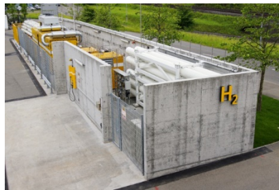
H 2 production used by fuel cell PostBus. Max. day production: 2500 nm 3 [3]
