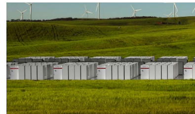
Tesla Powerpack in South Australia with 100 MW of capacity [4].
