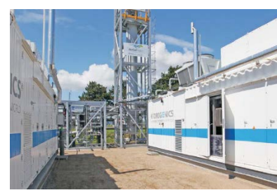
1MW of electricity is used to generate methane for gas grid [4].
