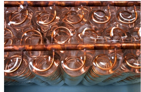
Ice forming around the heat exchanger coils inside an ice storage [1].
