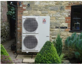
A 14 kW air-source HP for residential hot domestic water heating [1].
