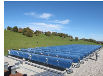
Collector field in industry (Parabolic trough collector)
