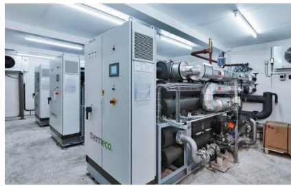
An 800 kW heating and 550 kW cooling system using 3 CO 2 HP in a slaughterhouse in Zürich (CH) [2].
