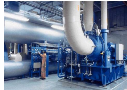
A 180 MW system of 3 HPs using sea water as heat sink for district heating in Värtan Ropsten (Sweden) [3].
