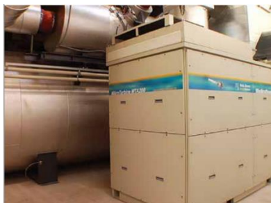
A 200 kW e cogeneration combined cycle gas microturbine in a food production plant in Naarn (Austria) [1].
