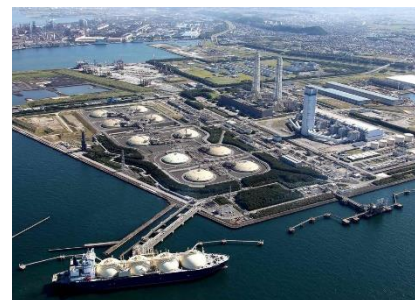
A 5'600 MW e power plant (21 GTs) using liquefied natural gas in Kawageo in Japan (Sweden) [4].
