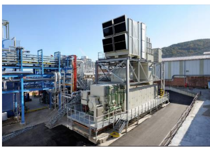
A 24.5 MW e natural gas combined cycle GT produces steam for a pulp & paper industry in Girona (Spain) [2].
