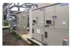
Kobelco has already installed some of their heat pumps in two factories in Japan. In Hokkaido Bioethanol Co. Ltd. where the heat pump is using the condensation of the ethanol gas as a heat source and creating steam for the distillation tower. In the company Meito Sangyo Co., Ltd. a similar process is also used where the steam is the heat source of their methanol distillation tower.
